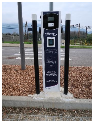
Borne Ingeteam 22/22 kW AC-AC
